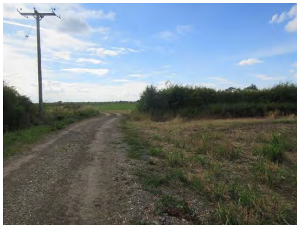
Photograph 20. Farm access track towards substation and transformer location which is on the right.. Negotiable with caution and confirmation of overhead clearances to power lines. New road construction to substation to be considerate of ALL loadings.
