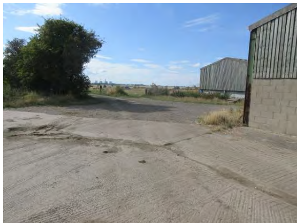
Photograph 15. Farm access through outbuildings. Load moves away from camera. Negotiable with caution and with courtyard kept free of vehicles and any other items that could be in store. Note there is a gradient here and change of level but this is negotiable by using trailer hydraulics.
