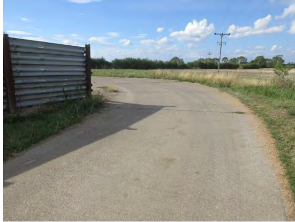
Photograph 10. Farm access track towards left hand turn. Load moves away from camera. Expected to be negotiable. Exact requirements to be confirmed once final loaded trailer arrangement known. Temporary plates on outside of the bend could improve turning radius or remove fence panel.
