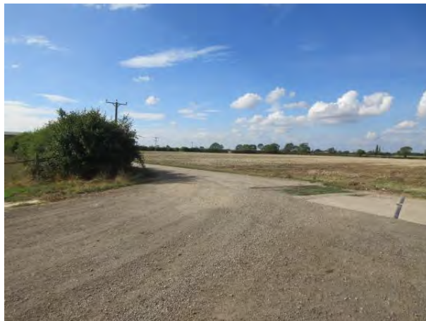
Photograph 6 First left turn on farm track. Load moves away from camera. Negotiable. Temporary road widening via plates or hardcore could be undertaken if required to widen road surface but this is not expected to be necessary..
